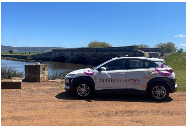
Above: Ross Bridge
